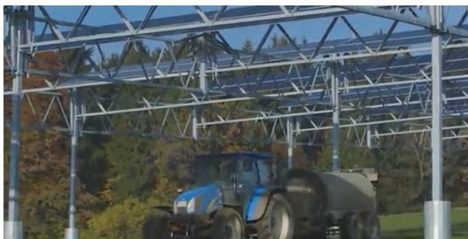
Figure 32: Example Agrivoltaic Installation
