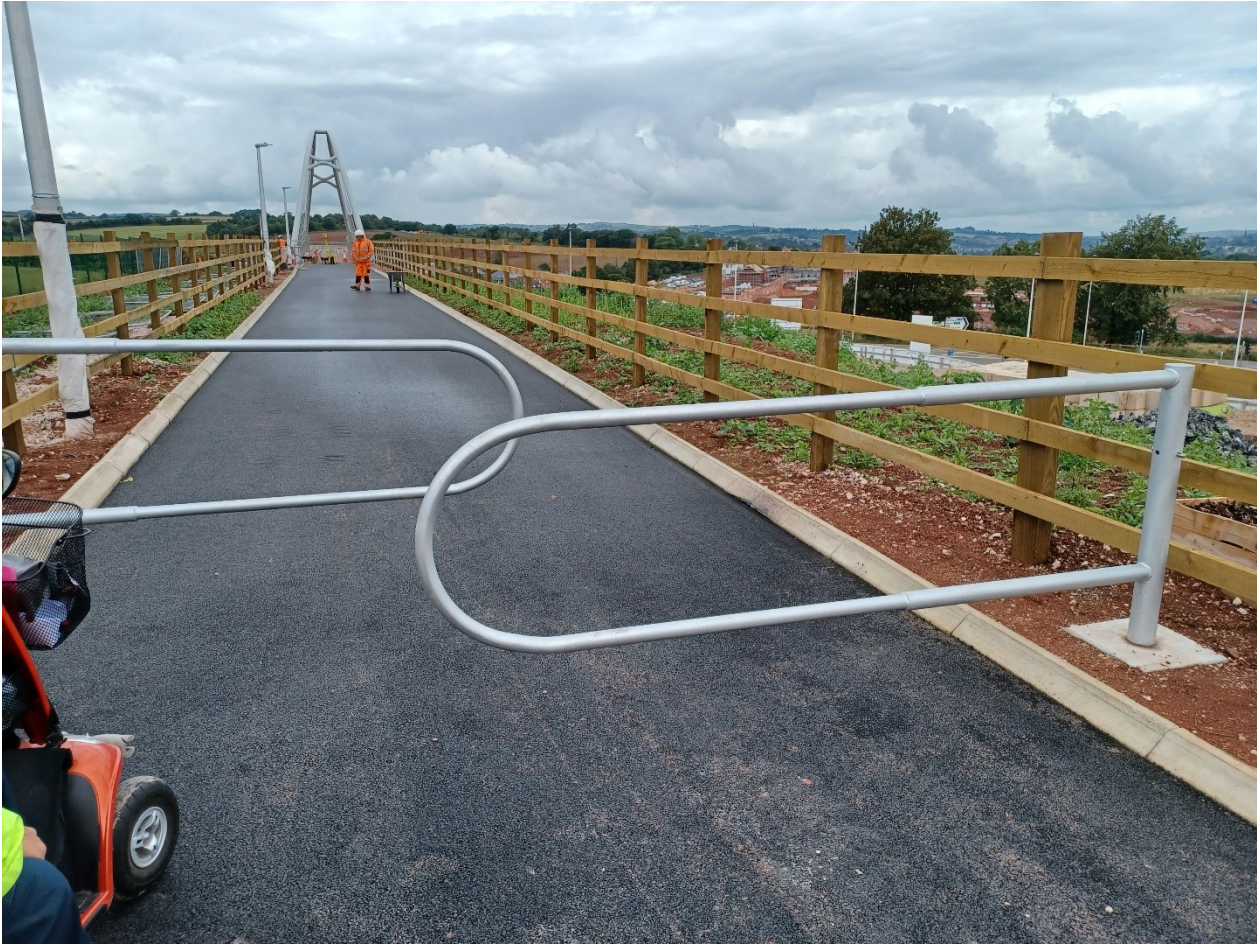
Photograph of chicane on A379 bridge, near Matford, Exeter
