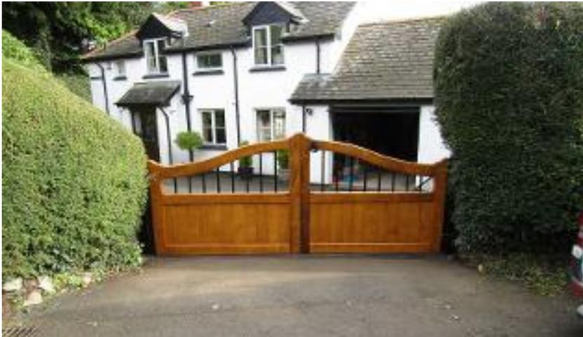
The scheme is utilising the EA's PFR framework with the contractor, Watertight International, utilising timber gates that are British Standard Kitemarked to give the village passive flood protection. Installation of the PFR measures is due to be completed prior to April 2022.
