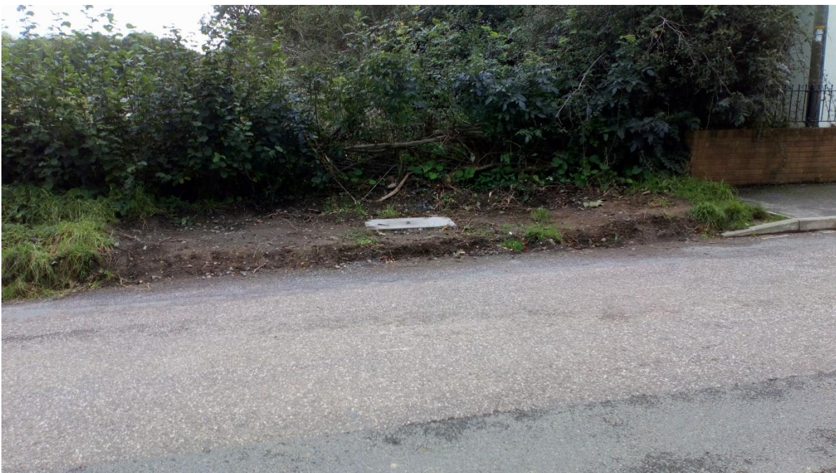
Photo – Lowered BT chamber in verge
