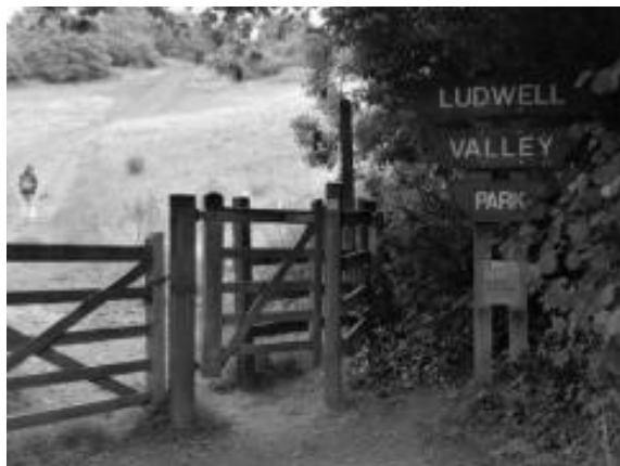
Inaccessible kissing gate
